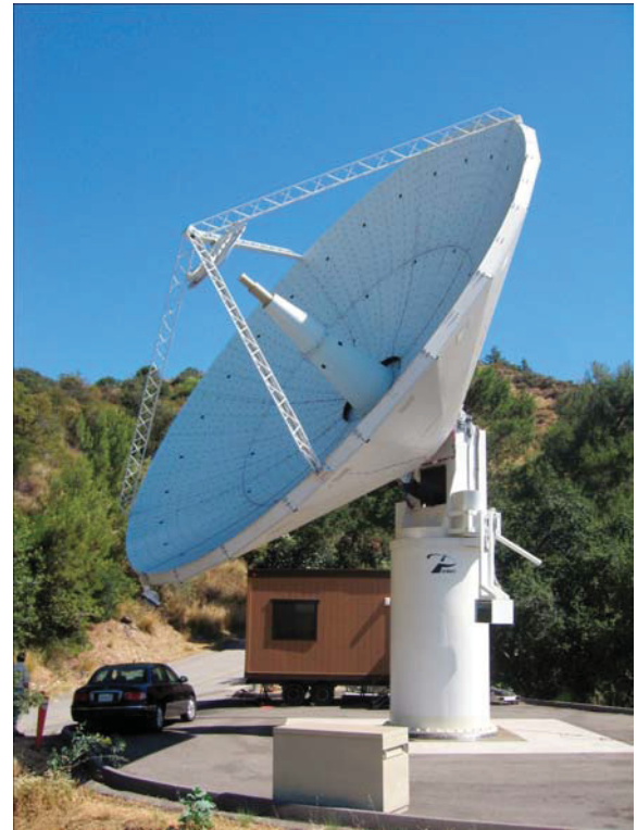
Fig. 4 The 12-meter dual reflector antenna
