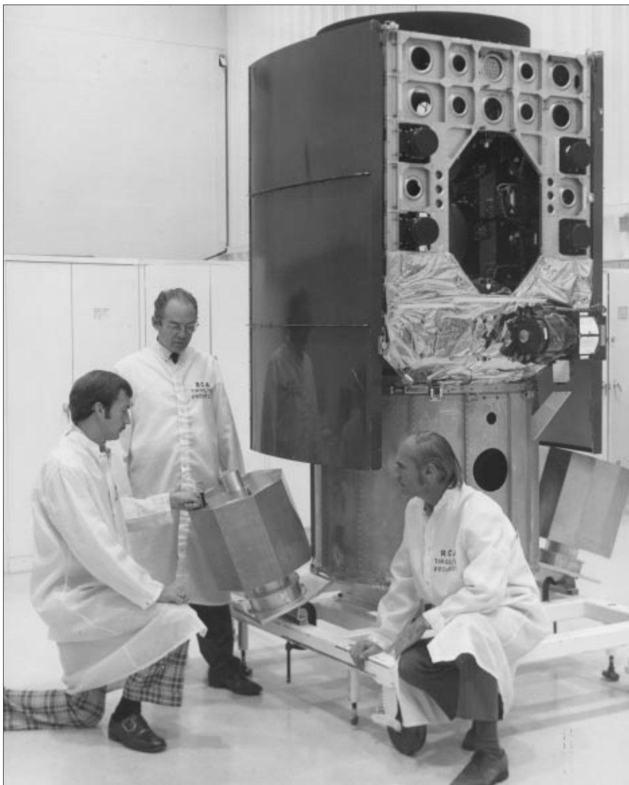
Fig 22-13 — The OSCAR 7 quadrifilar on its test model in its piggyback launch configuration alongside the flight-model ITOS spacecraft with which it flew. Left to right are Bricker, Maxwell (W2DU), and Ozman (W2WGH).
